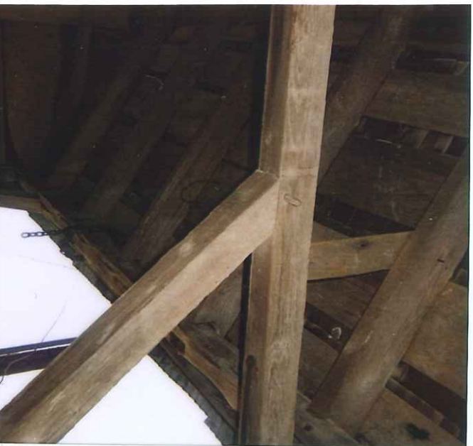
HAND CHOPPED TIMBERS IN BARN WITH WOOD PEGS
